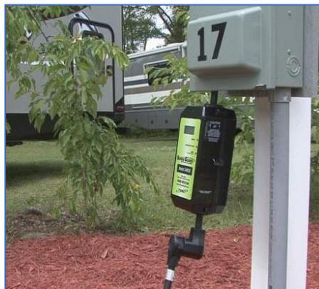
The Surge Protector connects the same way. The protector plugs into the park pedestal and your RV plugs into the protector. The electronics inside the protector analyze the voltage and wiring and decides if it is safe to connect your RV to the pedestal. **These devices are good to use and are not prohibited.**
