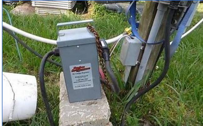
You generally would set them at the RV park power pedestal. The Autoformer power cord would connect into the pedestal power and your RV power cord would connect into the Autoformer. The original Autoformer only boosted low voltage on the RV parks power to your RV... the newer Autoformer now also includes a Surge Protector. **---these are the devices that are now prohibited---**
